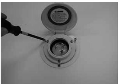
6. Position the gasket and inlet over the provided adapter mounting bracket, align the mounting holes and tighten the screws to 5-7 in.-lbs. torque with provided 8-32 screws. Fasten the mounting bracket to existing mounting holes.
