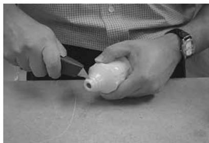
1. Cut boot at first line for cable greater than 10/3. Invert tapered end of the boot and apply soap solution.
