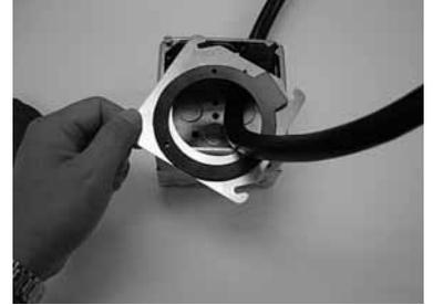
3. Pull out enough of cable to allow room to work. Tighten two screws of the box extender to the box with 10-12 in.-lbs. Feed cable through box cover opening and inlet mounting gasket.
