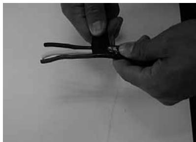
2. Remove 6" outer cable jacket and fillers. Use electrical tape to cover the jacket and flatten out conductors, leaving 2" exposed conductors. Feed conductors through rear safety enclosure.
