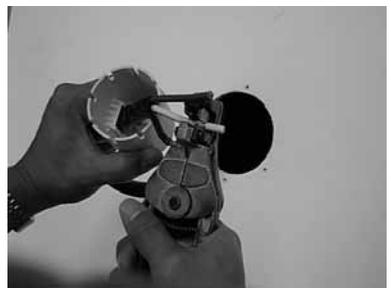
3. Strip wire ends 1/2" to 5/8". **Make sure the wire strands are clean and not corroded.** If necessary, cut back the wire until clean wire is uncovered. **Do not solder the ends of the wire.**
