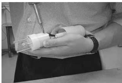
5. Insert bare wires into their corresponding color-coded terminals. Make certain there is no wire insulation under any terminal clamp. Tighten the screw clamps to 14-20 in.-lbs torque.
