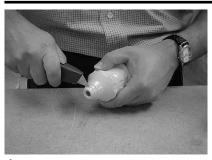
1 Cut boot at first line for cable greater than 10/3 (or greater than 5/8 in. Dia.).
