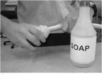
2 Apply soap solution to boot end and invert by pushing cord end against boot end. Push cord about 12 in. through boot
