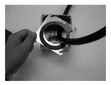
**3.** Pull out enough of cable to allow room to work. Tighten two screws of the box extender to the box with 10-12 in.-lbs. Feed cable through box cover opening and inlet mounting gasket.
