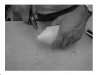
**1.** Cut boot at first line for cable greater than 5/8". Invert tapered end of the boot and apply soap solution.
