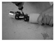
**6.** By alternating between two strain relief screws, tighten the screws to 14 in.-lbs. torque
