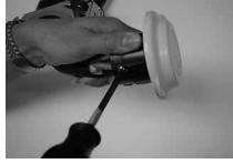
5. Back off terminal screws on the rear housing of the inlet. Insert wires into color coded openings on the back of the inlet. Tighten terminal screws to 22-25 in.-lbs. torque for 50 amp device. Make certain there is no wire insulation under any terminal
