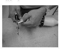
**4.** Strip outer jacket of cable 2" and 5/8" of insulation off each of the conductors. Cut away filler. **Make sure the wire is clean and with bright copper color.** If necessary, cut back insulation until clean wire is uncovered. **Do not solder the ends of the wire.**
