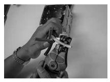
4. Remove 2" outer cable jacket. Strip wire ends 5/8" to 3/4" for 50 amp. Make sure the wire strands are clean and not corroded. If necessary, cut back the wire until clean wire is uncovered. Do not solder the ends of the wire.
