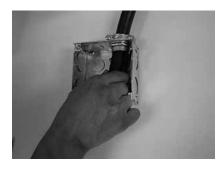
1. Unscrew J-box cover and cut off all wire connections.
